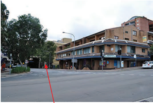
13. View to subject site from entry to cemetery.
